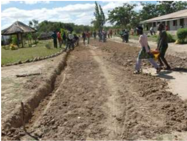
Digging for drainage
